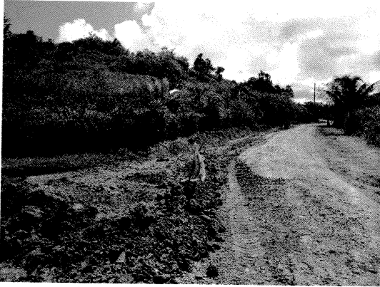
Pipe laying to Elechui
