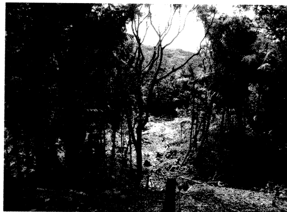
Clearing Area for Water Pump
