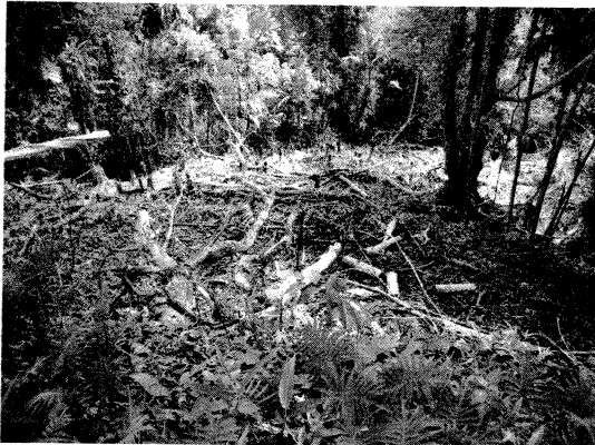
Clearing Area for Generator
