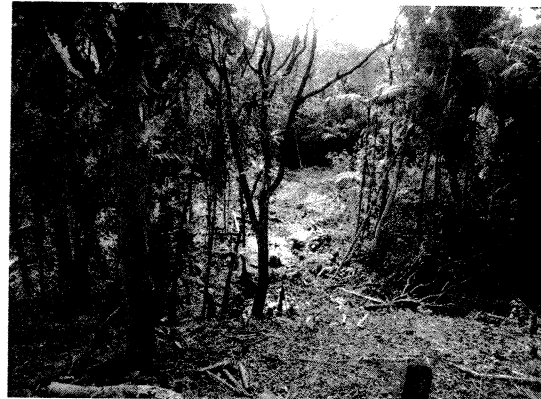
Clearing Area for Pump and Generator
