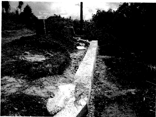
Water pipes to Elechui
