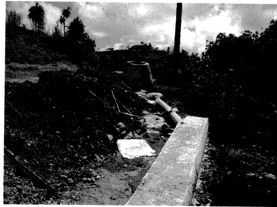
Water pipes and Manhole
