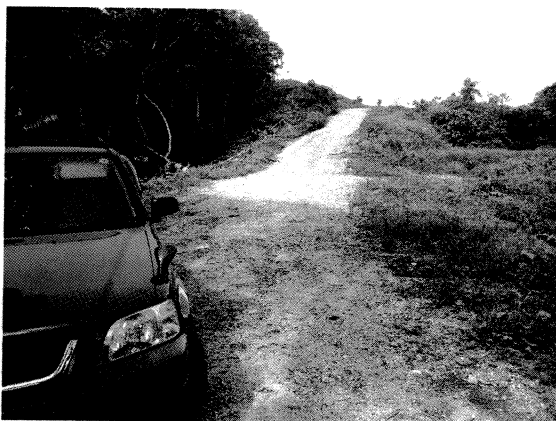
End of Access Road to Dam and Water Pump and Generator
